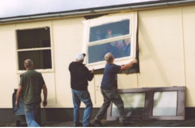
Demolition of the old classrooms underway.
