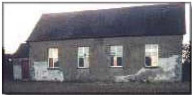
The partially renovated Free Presbyterian hall, at Annyart.
