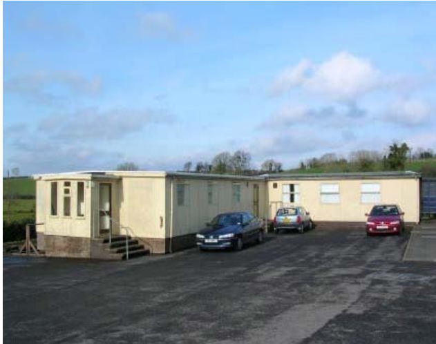
The classrooms in need of replacing
