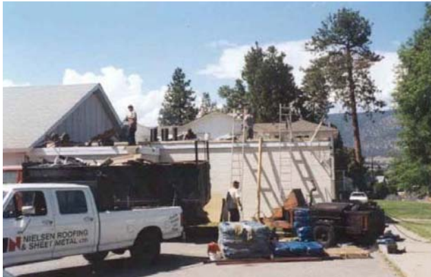
Repairs under way
